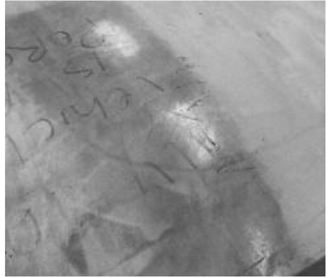
Figure 6 Detail of the damaged top end of one of the shell elements
